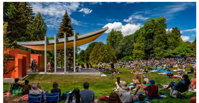
Volunteer Park Amphitheater, Seattle, WA Firm: ORA Architects
