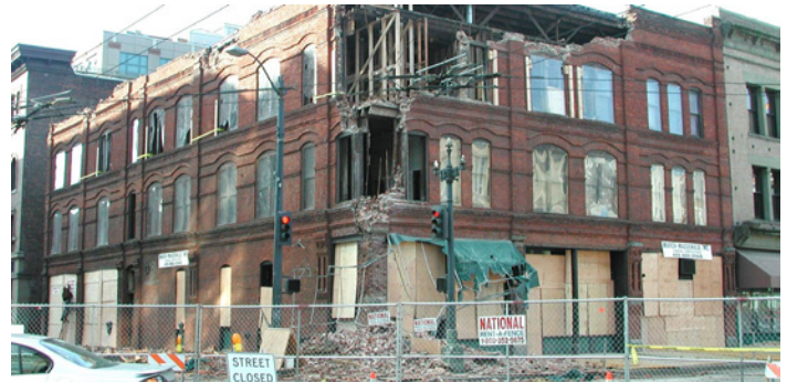
Nisqually Earthquake Damage to The Cadillac Hotel
